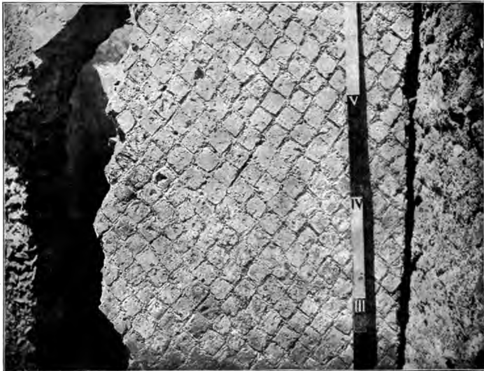
SPECIMEN OF OPUS RETICULATUM . 1
